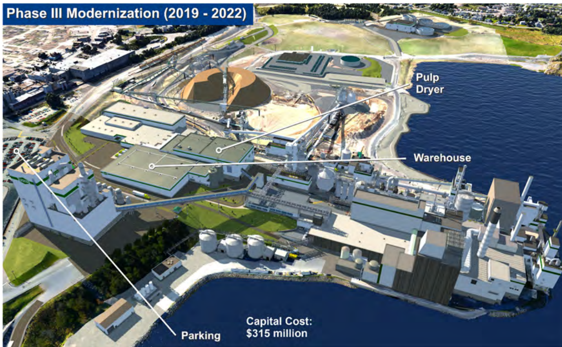
Figure 5. Three-dimensional model of the Reversing Falls Mill in Saint John, New Brunswick highlighting the Phase III Modernization completed between 2019 and 2022.
