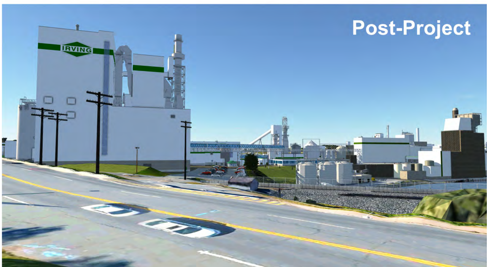
Figure 101. Modelled images showing the view of the Mill from Bridge Street at Mill Street before and after construction of mill modernization and green energy generation project at the Reversing Falls Mill in Saint John, New Brunswick.
