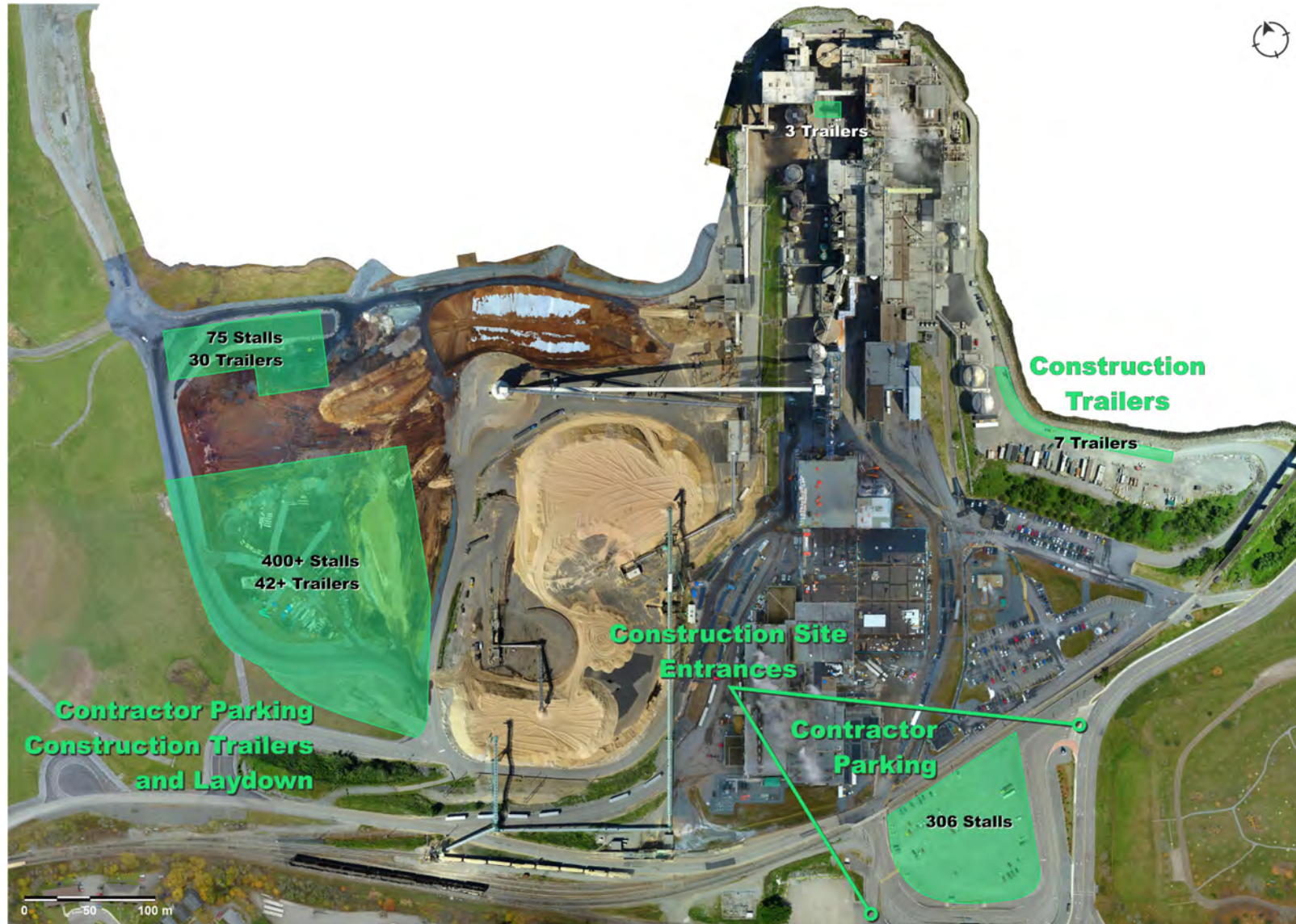
Figure 34. Aerial photograph of the Reversing Falls Mill, circa 2022, in Saint John, New Brunswick showing construction and parking areas and entrances for construction of the Phase IV Mill Modernization project.
