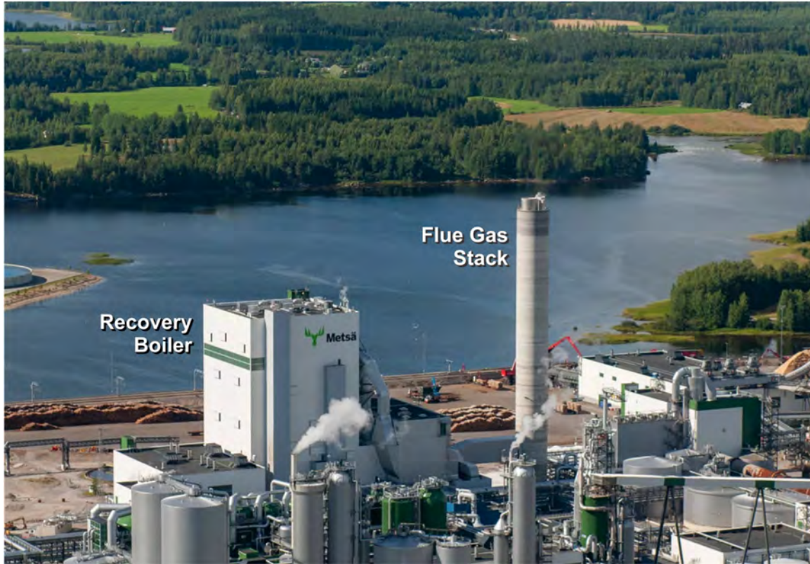
Figure 26. Photograph showing daytime operation of the recovery boiler flue gas stack at the Äänekoski bioproduct mill in Finland. Source: Metsä Group website.
